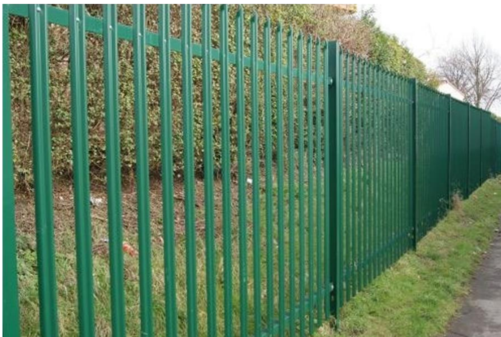
Plate 4.14 Typical Palisade Fencing
