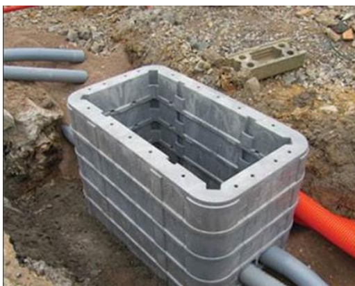
Plate 4.12 Fibre Chambers (construction and external appearance)
